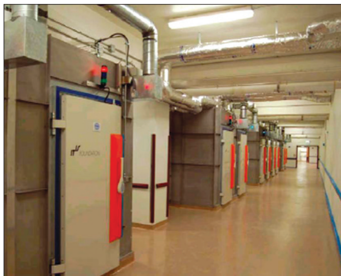
Chambers at the IIT Research Institute in Chicago where the studies took place.
